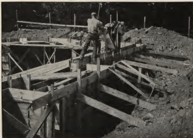
Forms for high concrete walls must be adequately braced to assure straight, plumb walls.
